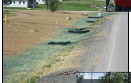
The contractor observed no problems or failure of the Flexterra-FGM, even though there was a rain event within one hour after the application. Stability was also maintained during the following 9 rainy days and there was no problem with sediment movement or brown water due to the addition of the Terra-Tube .
